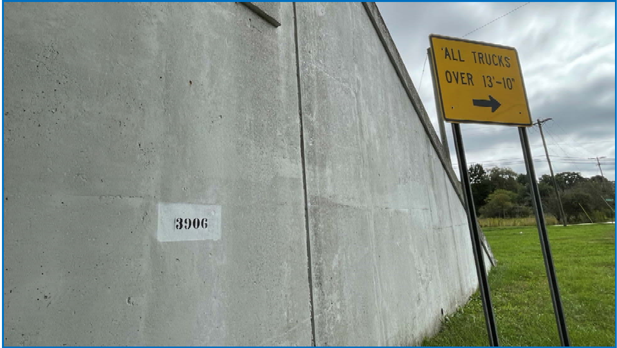
Photo 23: Wingwall 2B showing bridge number and vertical under clearance sign.
