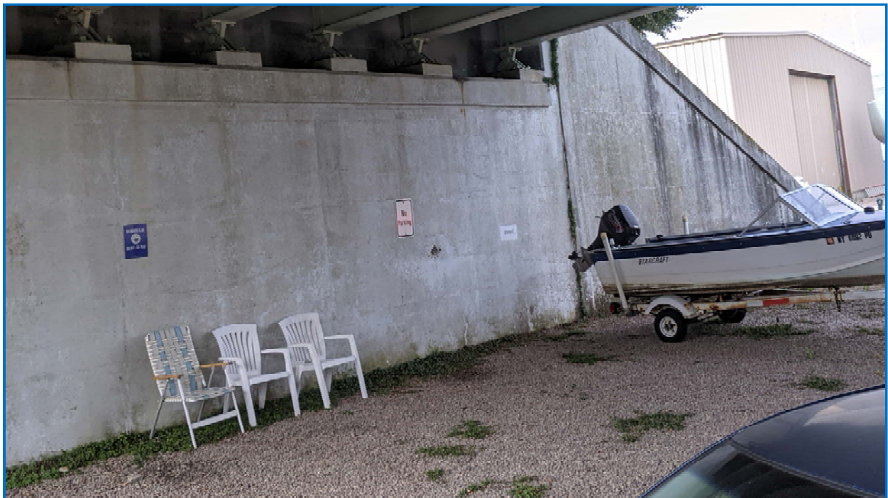
Photo 18: Abutment 1 and Wingwall 1A adjacent to Matthews/Main Street.
