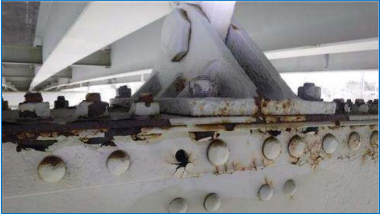
Photo 13: Typical condition of fixed rocker bearings.
