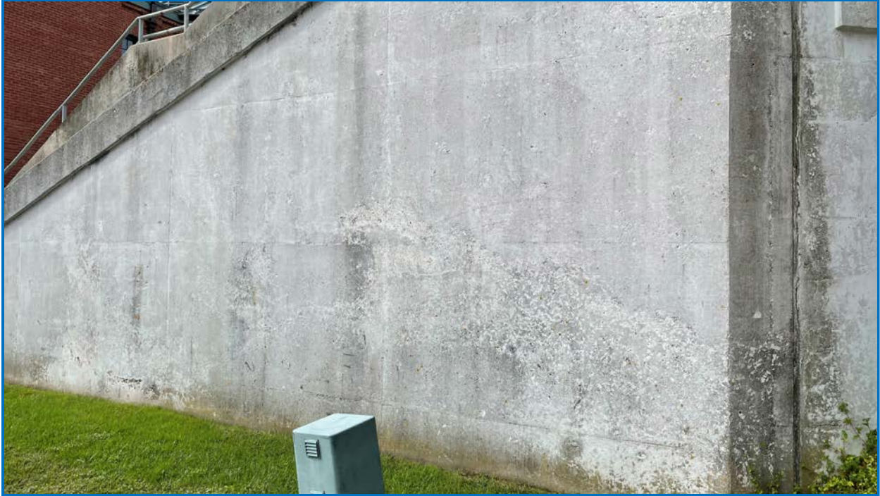
Photo 19: Wingwall 1B adjacent to stairway.
