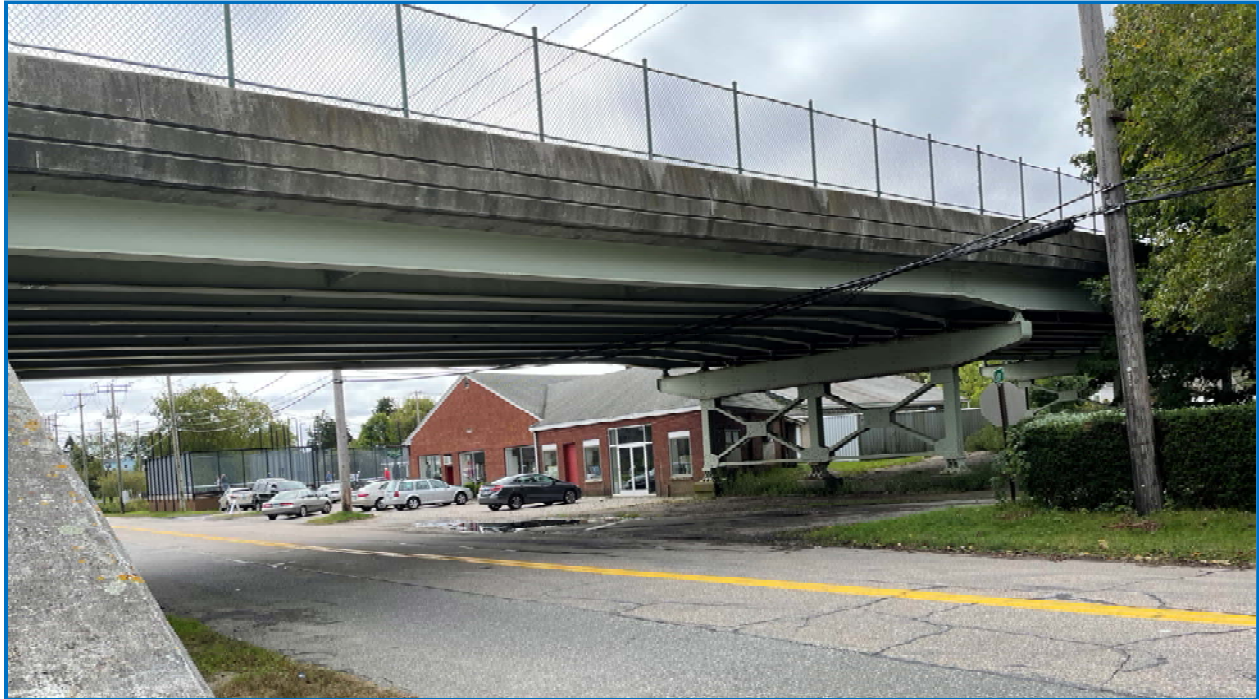
Photo 4: West elevation of bridge over Culter Street.
