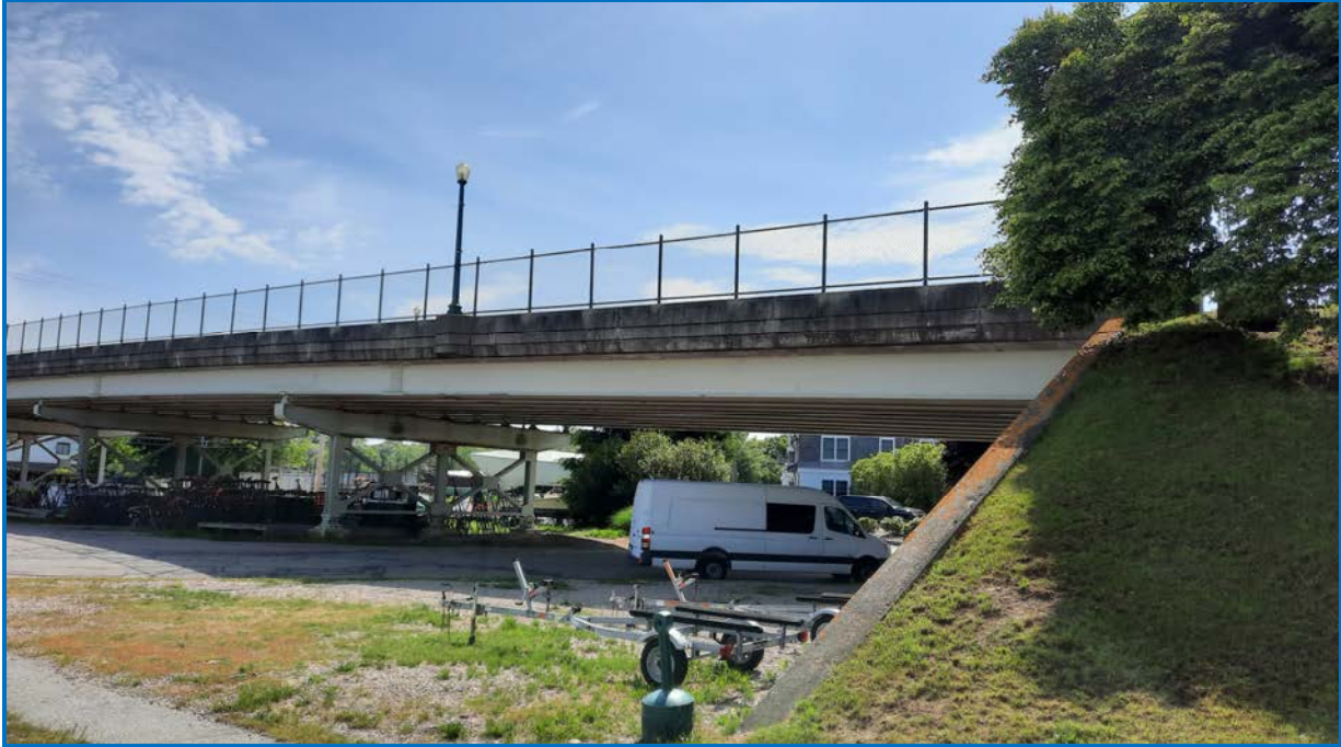
Photo 1: West elevation of bridge over Matthews/Main Street
