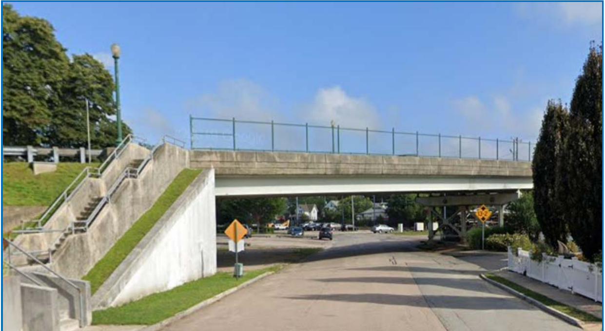
Photo 2: East elevation of bridge over Matthews/Main Street
