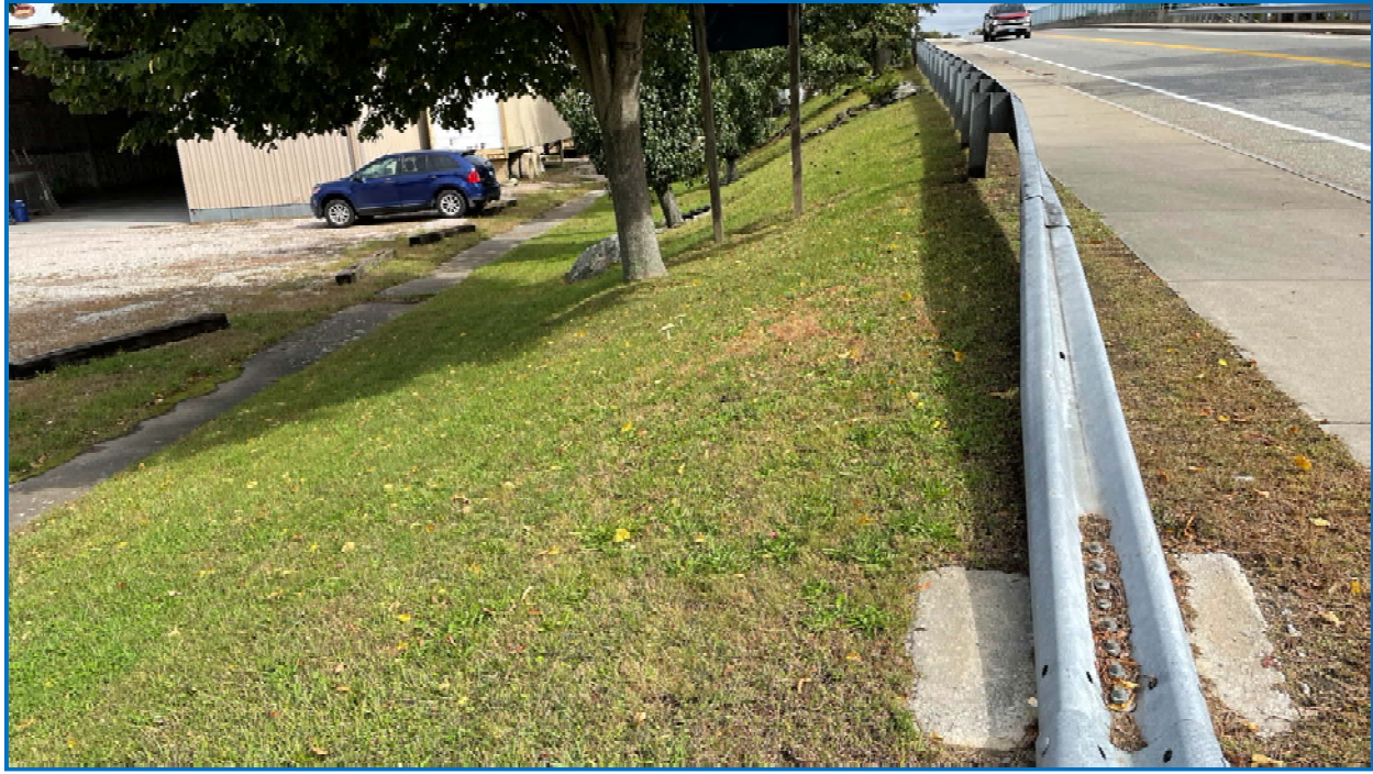
Photo 34: Guiderail end treatment and southwest approach embankment.
