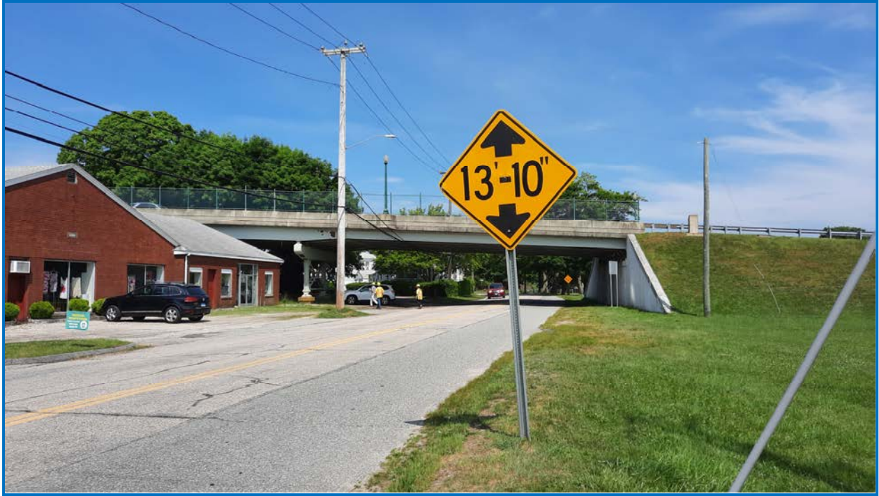
Photo 3: East elevation of bridge over Cutler Street.
