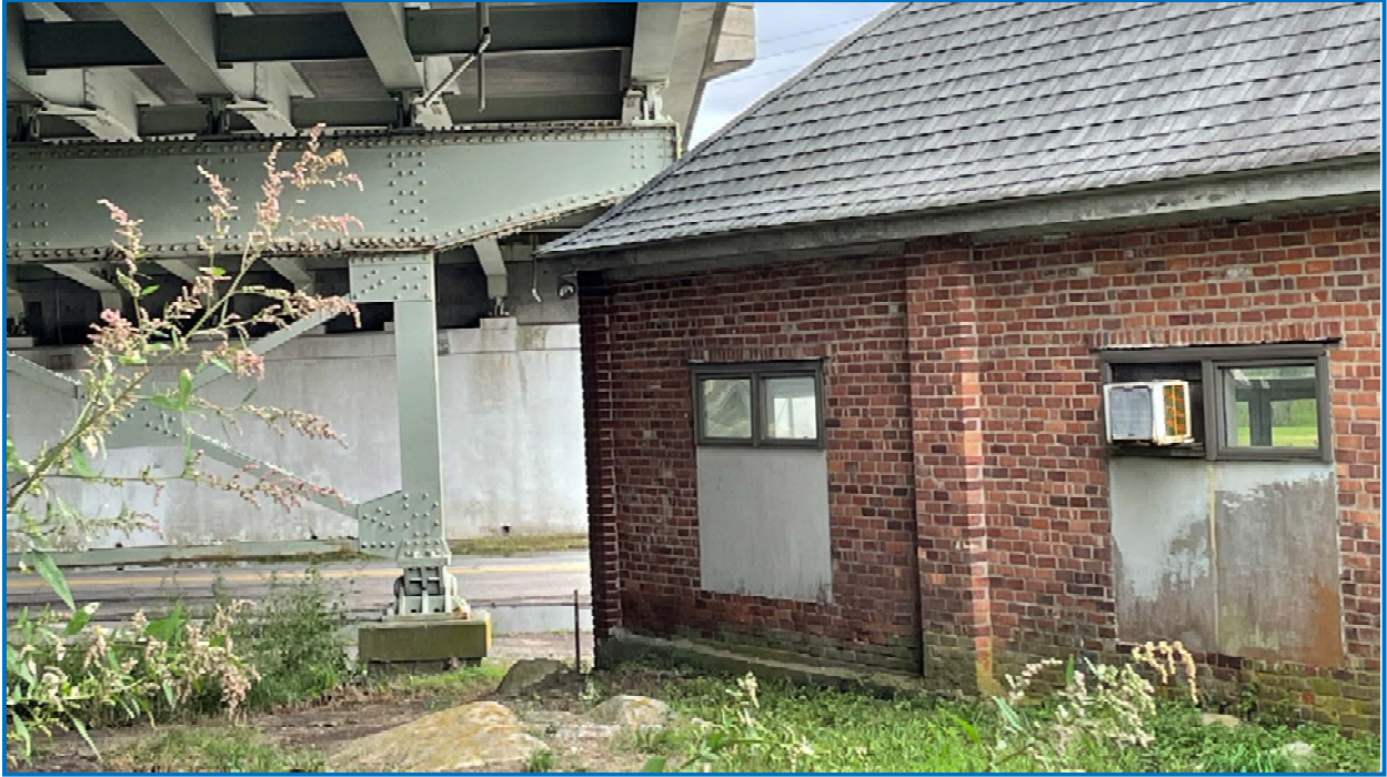
Photo 35: Portion of existing building located under span 7 and pier 7 (looking North).
