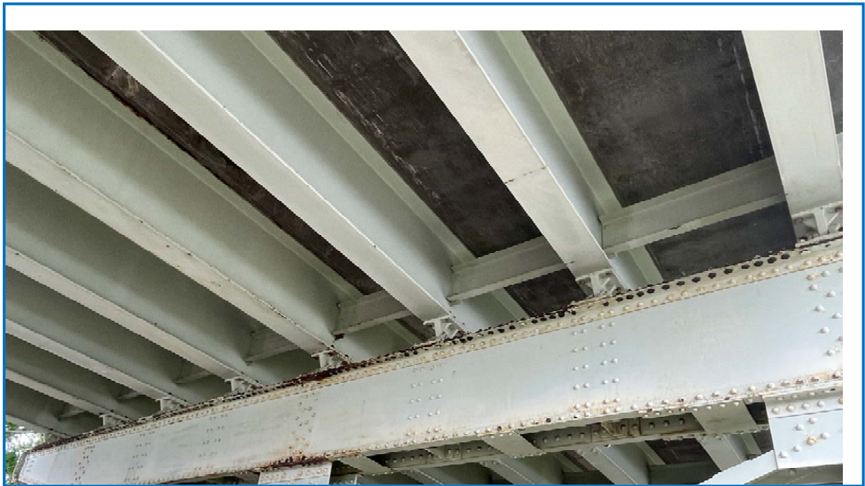
Photo 24: View of Pier Cap 6 from south side.
