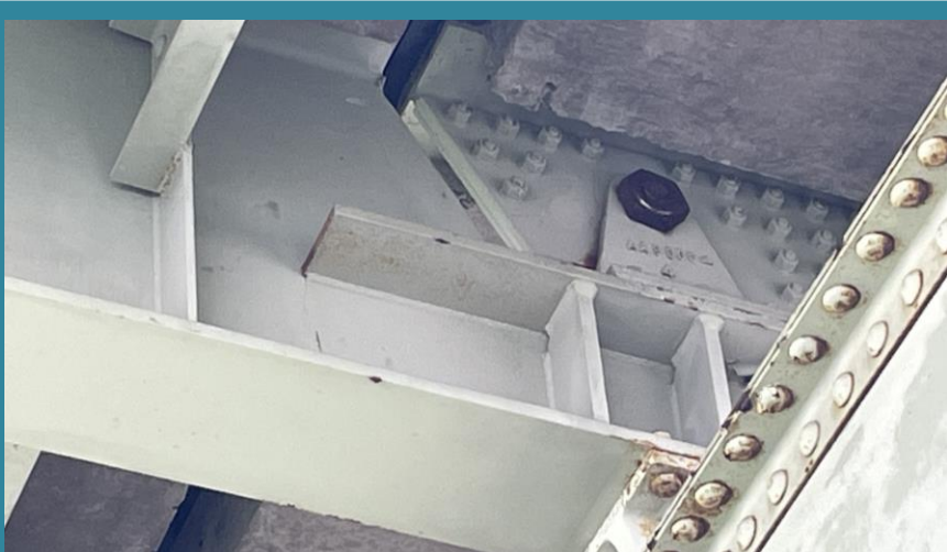
Close up of expansion bearings over Pier Bent 4.
