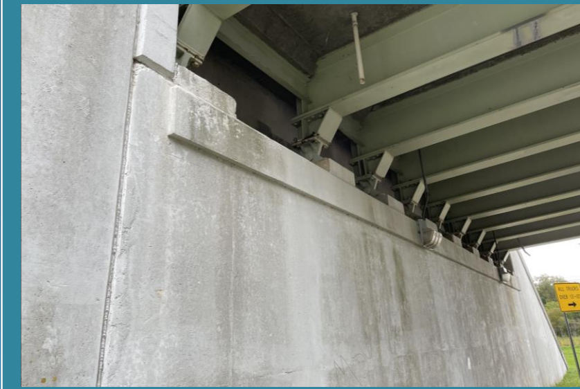
Abutment 2 adjacent to Cutler Street. 13'-10" vertical under clearance sign.
